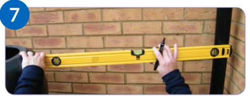
Use a level, positioned at the bottom of the your drilled hole.
