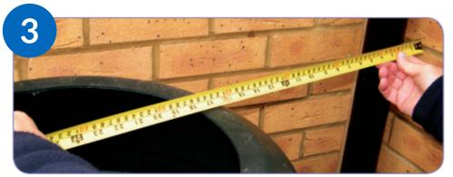
Make sure that the water butt is positioned no more than 500mm from the downpipe.
