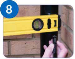
Mark a level line from the bottom of the hole on the downpipe.
