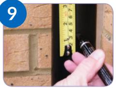
Mark 30mm/38mm/70mm\* above the level line on the downpipe.
