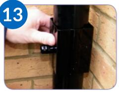
Manoeuvre the diverter onto the downpipe.
