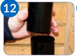
Remove the cut section.
