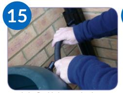
Attach the flexible hose to the diverter.
