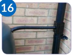
Attach the flexible hose to the water butt connector.
